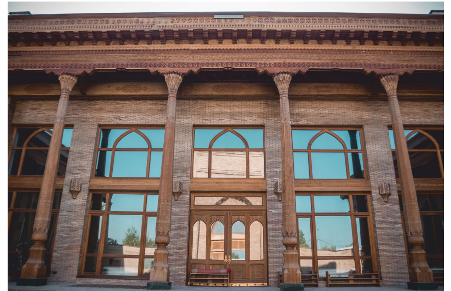
Columns and a roof with carved patterns created with the participation of Akmal Azlarov.
